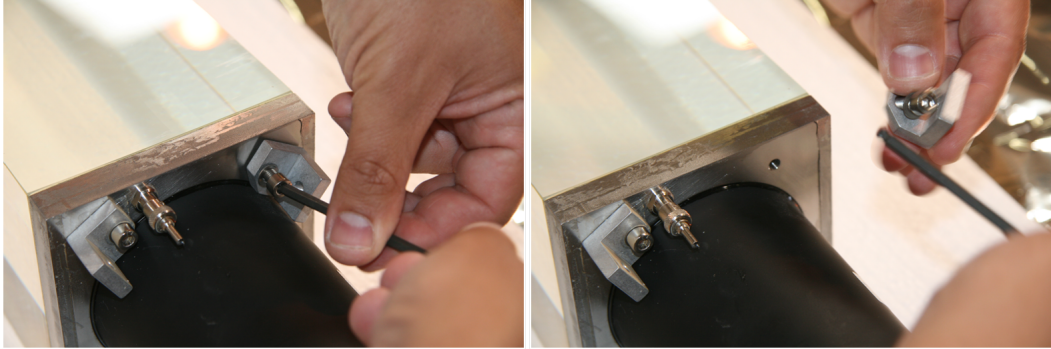
Figure 3.15: Steel flange with support bracket.
