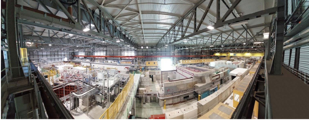
Figure 3.16: Picture of the EHN1 hall from above.
