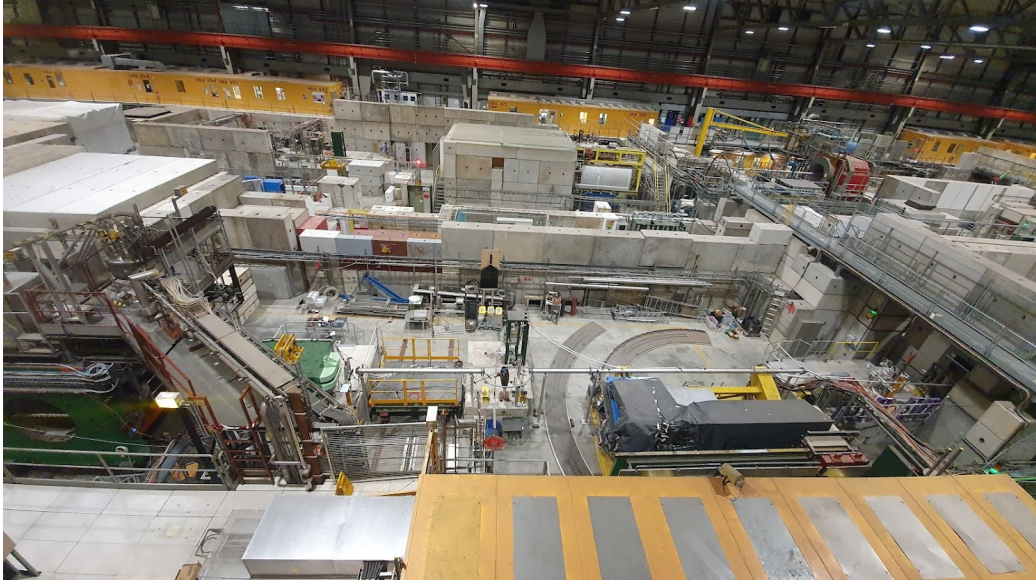
Figure 3.17: The PPE172 zone of the North Area H2 beamline, viewed from above. In the picture, the beam goes from right to left.
