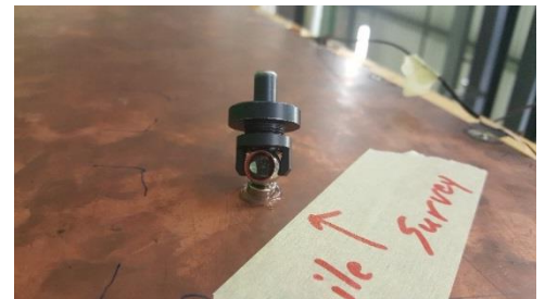
Figure 2 Survey point on the MM-DW
