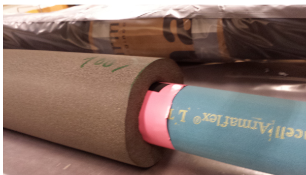
Figure 3.42: Photo taken during the assembling of the transfer line. In blue is the cryogenic type LTD, ID/OD 22/25 mm and gray the halogen free type, ID/OD 75/25 mm.
