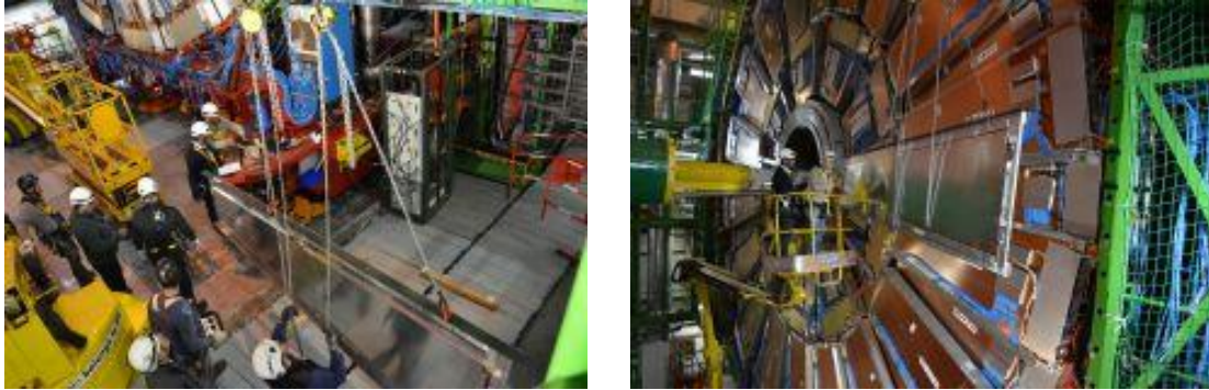
Figure 5.43: Lifting and positioning the first Super Module for the RE negative disk.
