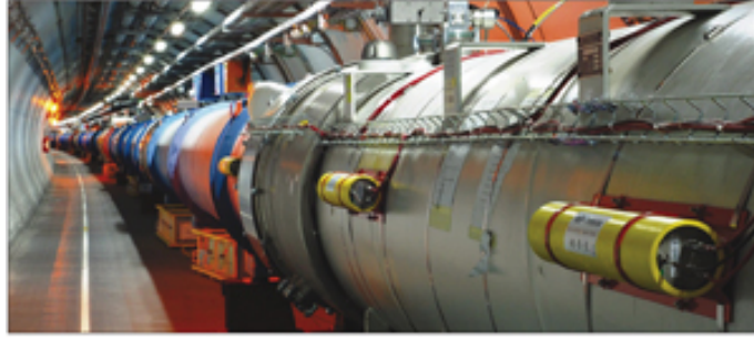
Figure 2.9 The location of the BLMs outside the cryostat in the LHC tunnel.
