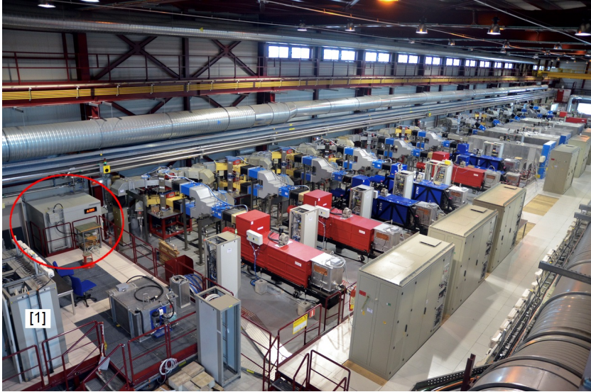
Figure 6.3: Laser cabinet (marked in red) situated above 160 MeV area of the LINAC4 tunnel and next to klystrons which supply the RF-cavities in the accelerator tunnel below this hall. [1] refers to the rack where the DAQ and control system is located.
