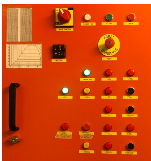
Figure 34 – Interface of TRACI CO 2 plant
