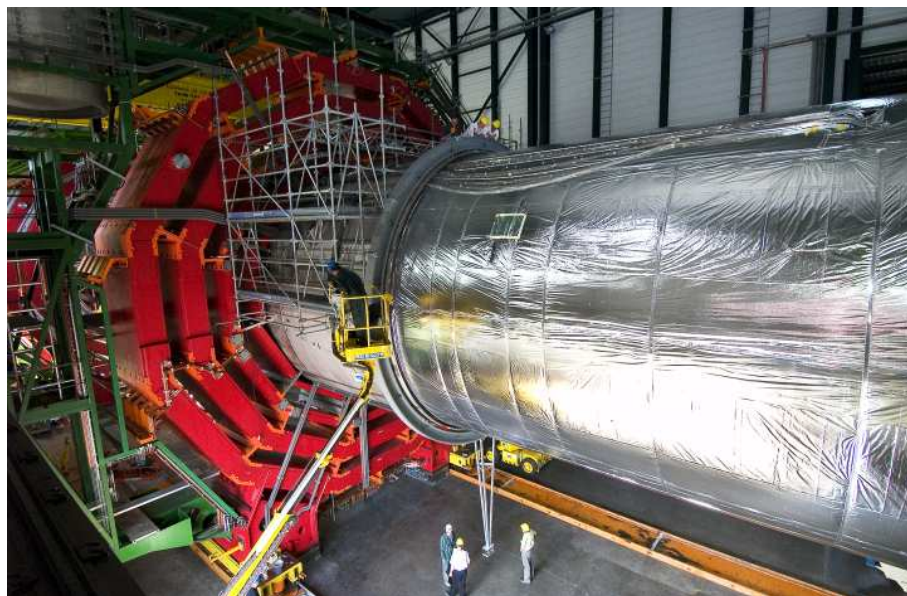
Figure 2.13: Insertion of the CMS solenoid magnet into the cryostat barrel during September 2005. As the solenoid was assembled in its vertical position, before the insertion it had to be swiveled to its horizontal position.
